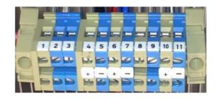
Terminals 4, 6, 10 and terminals 5, 7, 11 are bridged in the delivery status. To switch between cooling- and heating operation remove the bridges and connect a suitable controller, e.g. SCC-003-A.
